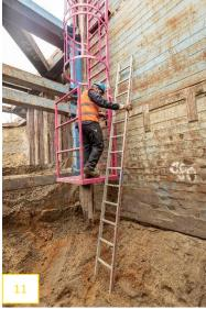
11 Depending on the landing side of the ladder on the lower platform, a chain is released on the right or left with carabiners.
