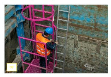
08 The ladder is attached tot he scaffolding by means of a chain, as tight as possible, around the ladder beam. This is to prevent tipping tot the side.
