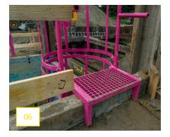
06 The ladder must lie completely on the surfae, in a suitable and straight manner.
