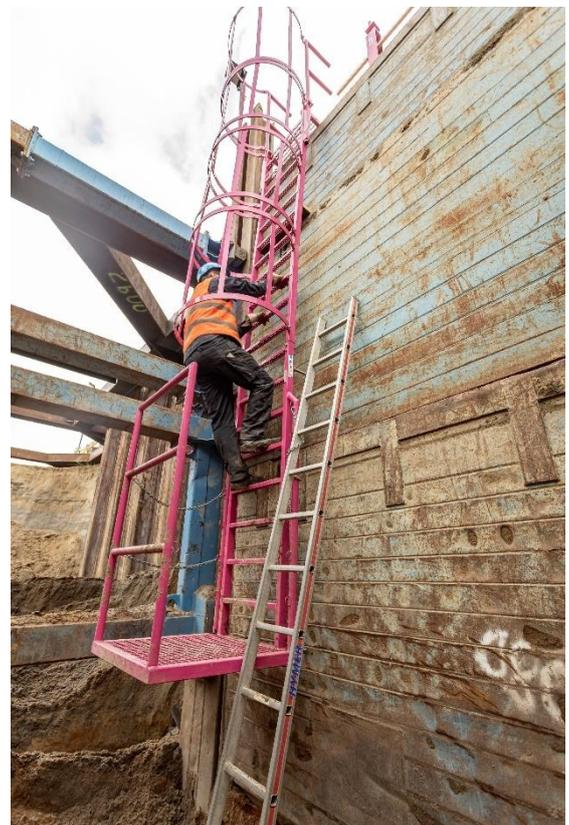
**Note:** For safety, clean shoes for walking up and down the ladder. Top and bottom grilles have been made for this purpose.
