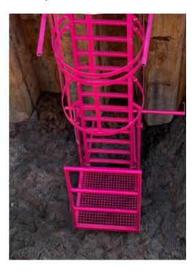
Depending on the correct position, the height of the cross pole is adjustable. The ladder part can also be secured with a chain to prevent slipping.
