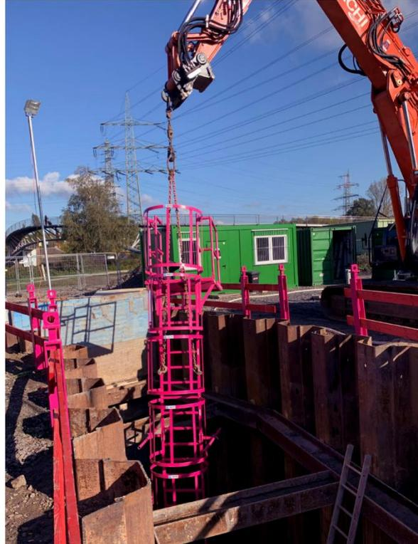
The 2 anchor points for attaching lifting chains are located on the top platform.
