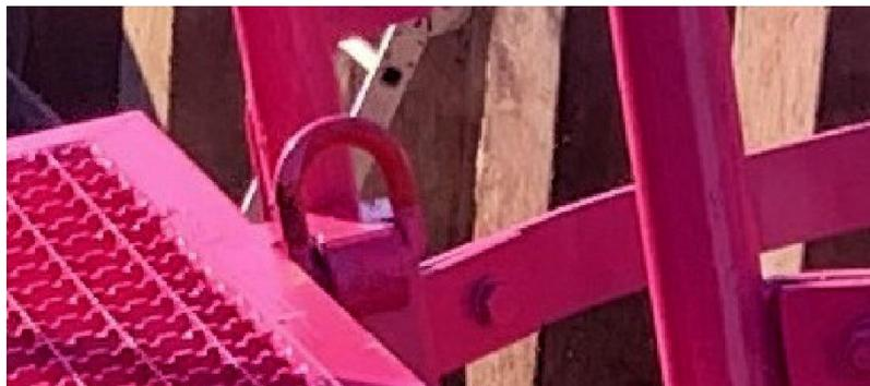
Once the top platform is in place, the mounting bolts should be drilled into the holes. Secure with split pins.
