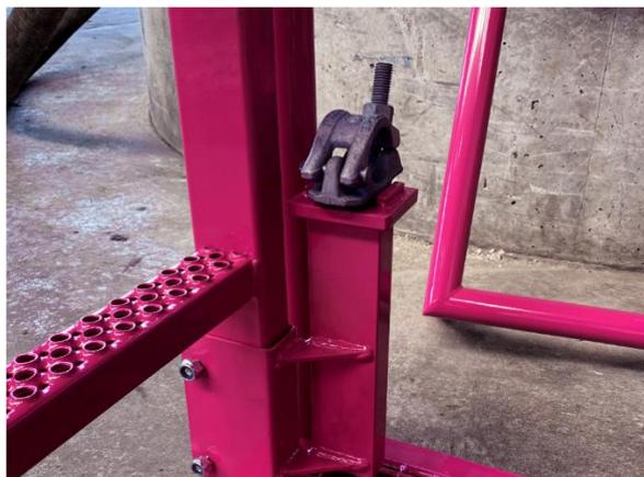
The bottom holder must be screwed 180 degrees and at the bottom. This is so that the support posts can be attached.
